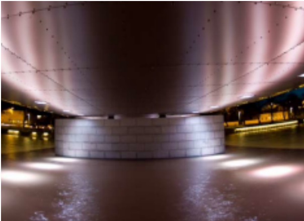
Molybdenum-containing stainless steel (grade 2205) cladding of the Myllysilta Bridge
