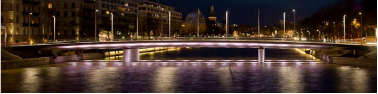
Myllysilta Bridge, Turku, Finland
